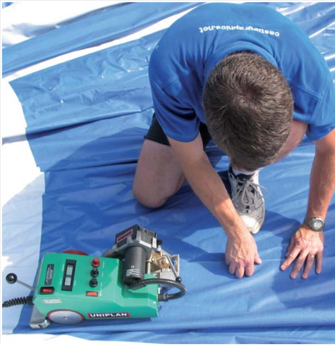
Joining the quadrants with the UNIPLAN E.
