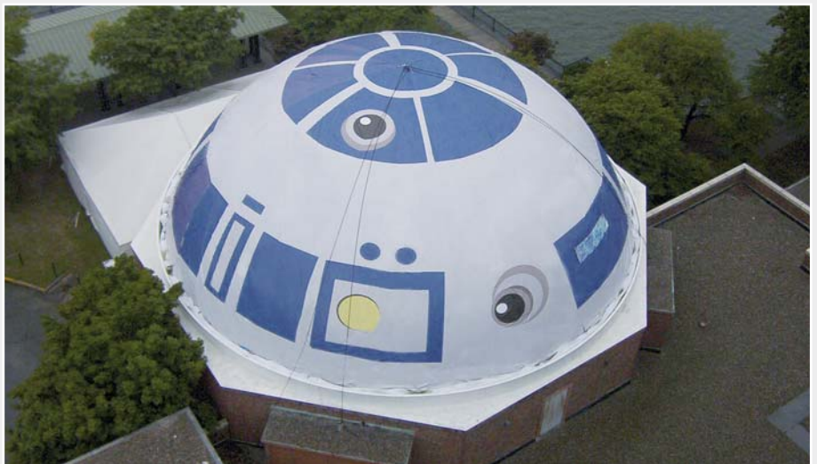
The finished R2D2 dome with a 197-foot circumference.
