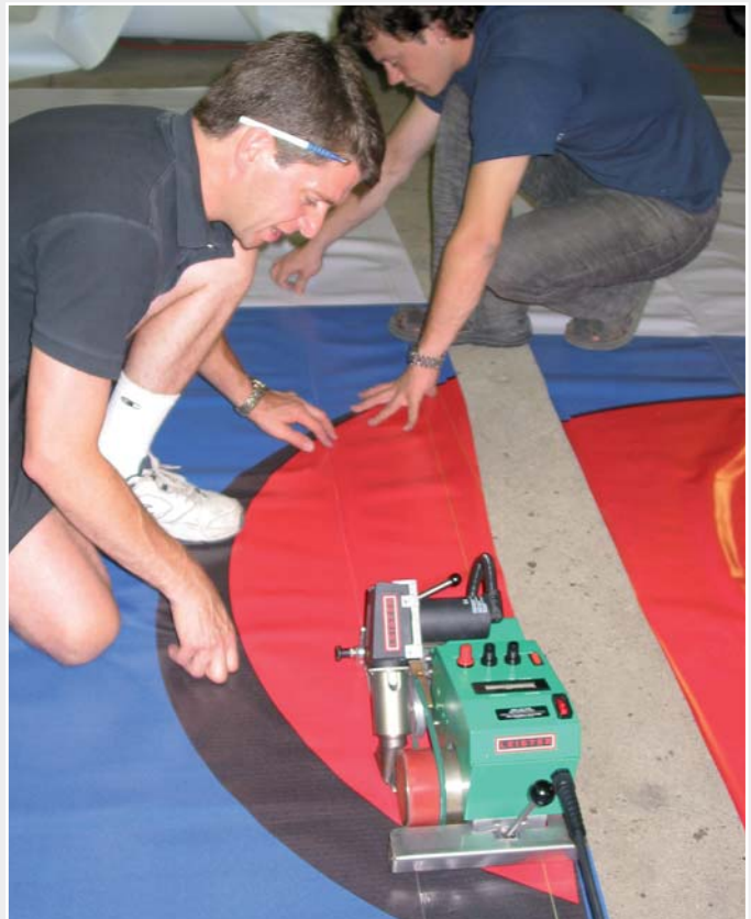
David King tailoring in the installation bay.
