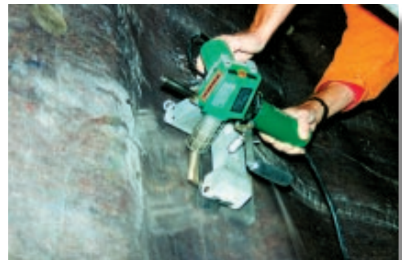
TWINNY S with combi-wedge short welding in a tunnel.
