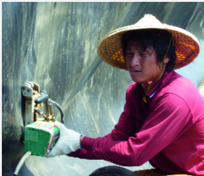
Welding of the HD-PE material on steep embankments with the COMET.
