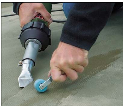
Welding waterproofing liners, tarps & tents
